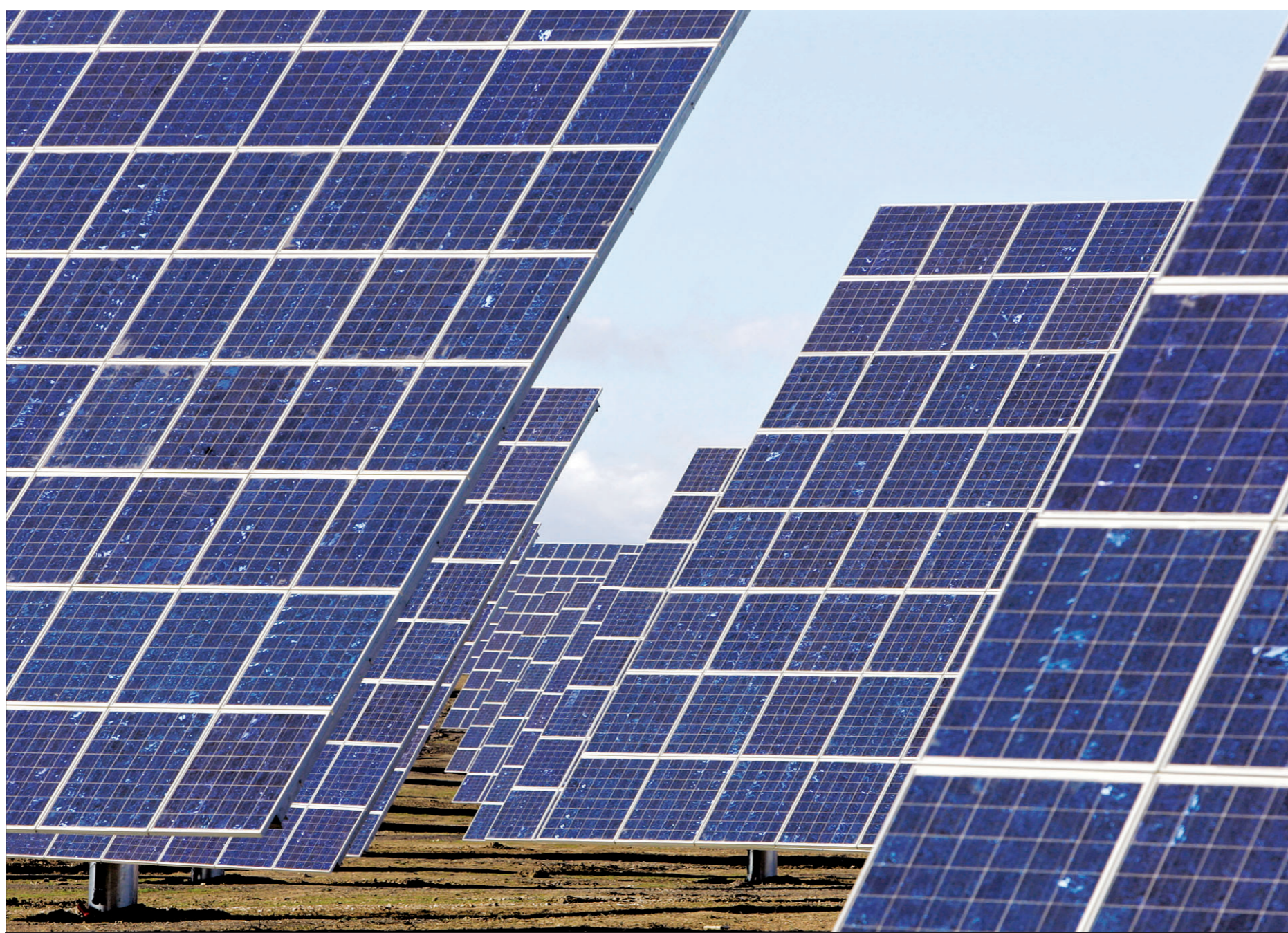
Sunbathing: the world's largest photovoltaic plant, consisting of more than 240,000 solar panels, is under construction in southern Portugal
